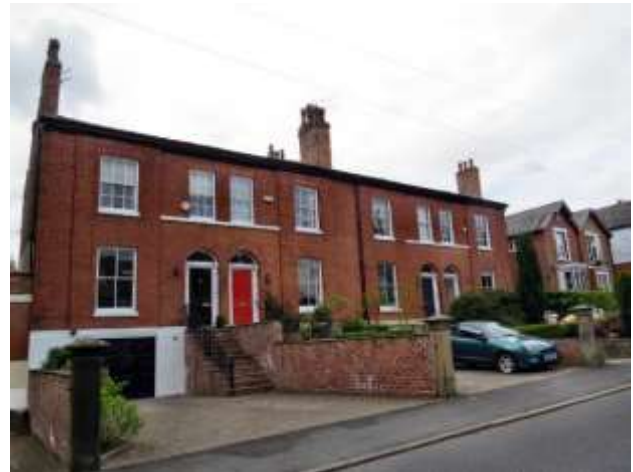
30-36 Stamford Road - a balanced classical terrace but with a harmful basement extension and front drive
