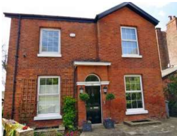
Detracting replacement uPVC windows in a mock-Georgian style, Langham Road
