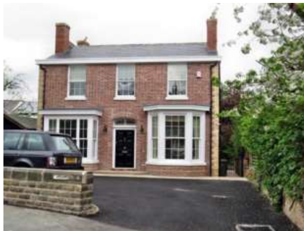
New development on New Road, which lacks any soft landscaping
