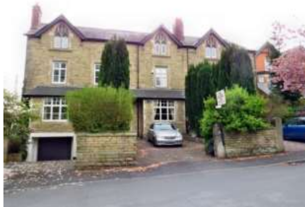
Substantial re-landscaping for the provision of a basement garage which has resulted in the elongation and mis-balance of the main elevation, West Road
