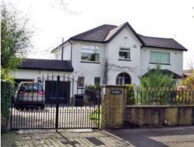
Inappropriate replacement windows on Delamar Road
