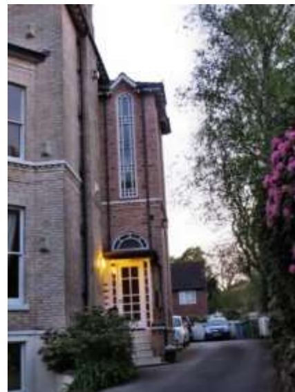
A good example of sympathetic alterations for the conversion of a building into flats, Heald Road
